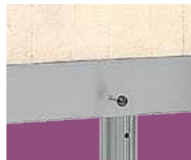
✓ Supply air bottom valve
